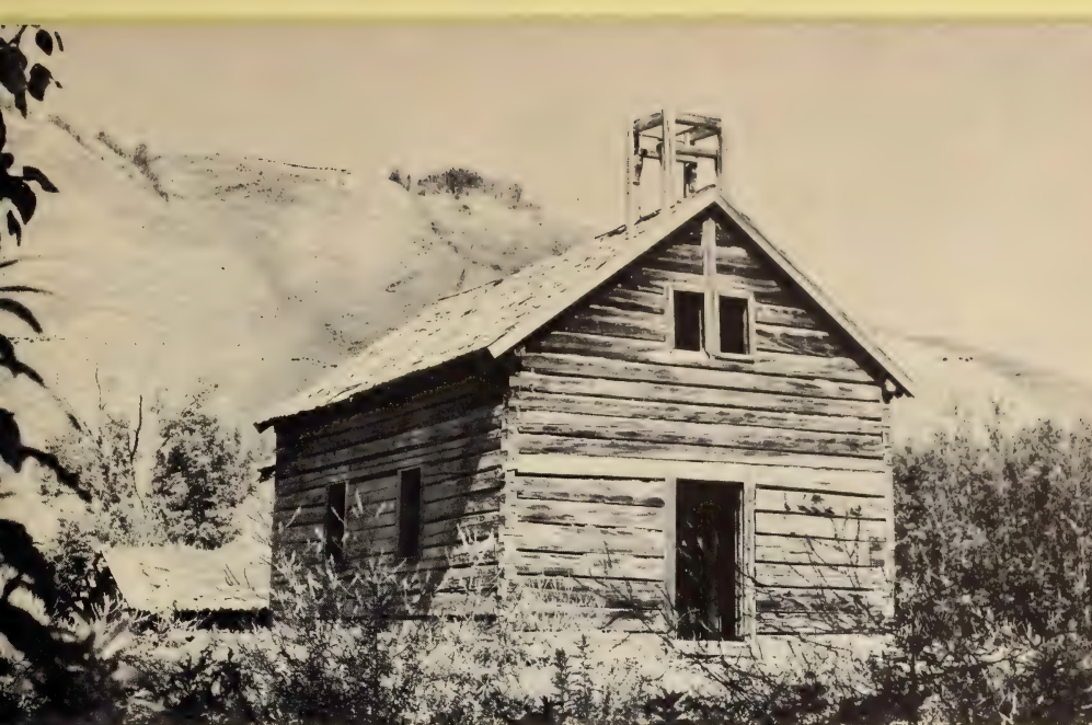
Grouard church is located in the scenic valley of the Peace River at Dunvegan Crossing, and played a vital part in the early missionary work of the area.
